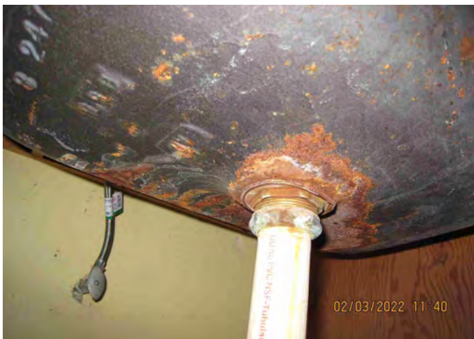
5.13 - The underside of the metal laundry sink is excessively rusted and the sink will need to be replaced. Note: The sink appears to be actively leaking at this time.
